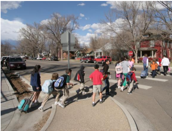
Figure 2. Curb Extension. Source: www.pedbikeimages.org/Dan Burden
